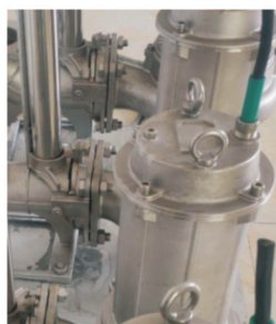
Booster pump 增压泵
